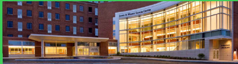
University of Rochester: EcoStruxure™ ensures reliability and saves several hundred thousands of dollars
